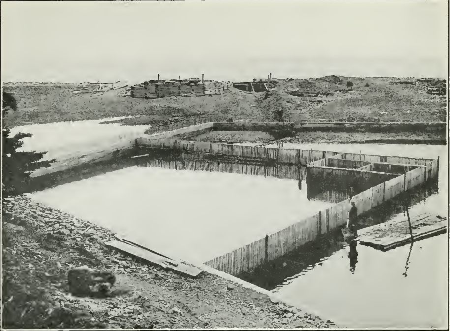
Fig. 1.—A mating pond with one large compartment and three smaller ones, all within the cement pond. The deepest water in the cement pond is immediately under the three small wooden compartments. This view was taken at about half tide, and shows the eastern side to be already bare of water. The man standing on the wall at the far side marks the position of the intake pipe.
