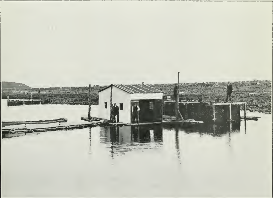
Fig. 2.—The plant viewed from the southwest side. A floating walk connects the engine house with the shore. The tall piles hold the rafts in place. The sea-wall is seen in the background.
