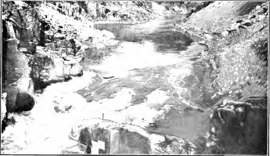
After completion of work—Note the eddy above the Gate in which the Salmon rest after going through the gate.
