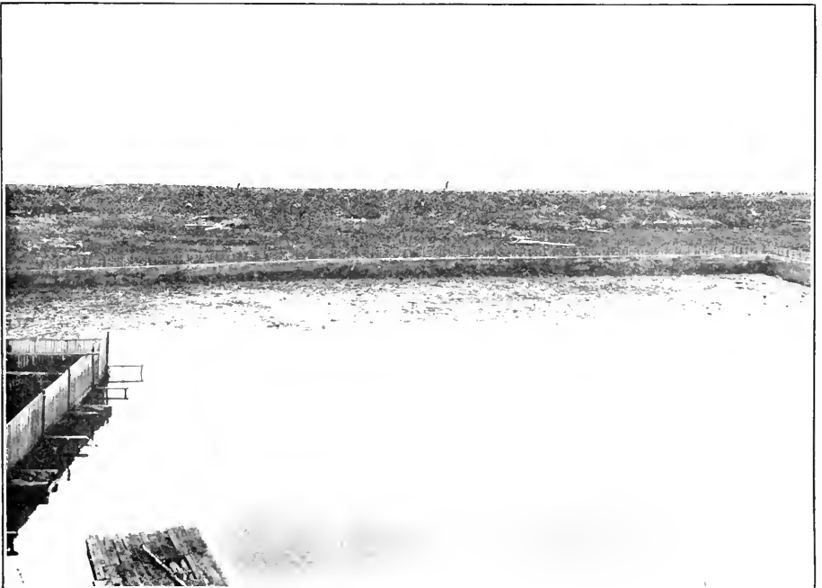
Fig. 2.—View of the eastern side of the cement pond taken near low tide. Nearly one-third of the bottom is bare of water. The rest is covered with water varying in depth from an inch to ten or fifteen inches. A small part of the wooden pond within the cement pond is shown at the left. The sea-wall is some distance beyond the cement pond, and St. Mary's bay in the background. The distant shore of the bay is faintly visible.
