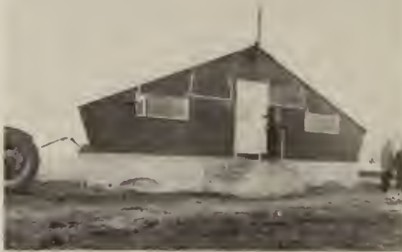
The new feeder hog building.
